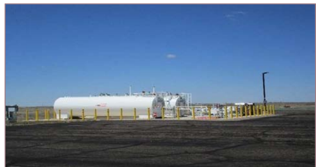
100LL and Jet A Fuel Tank and Self-Serve Fuel Station
